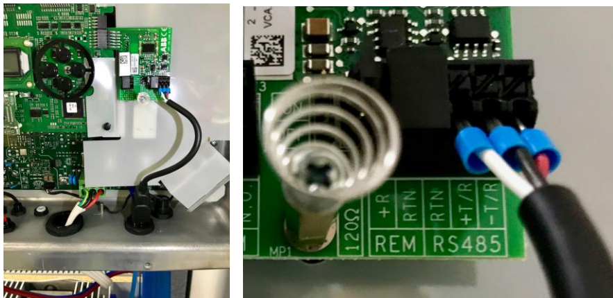
ABB UNO Connections (inside unit) – RS485 Adapter Wires terminated into the ABB communications board
